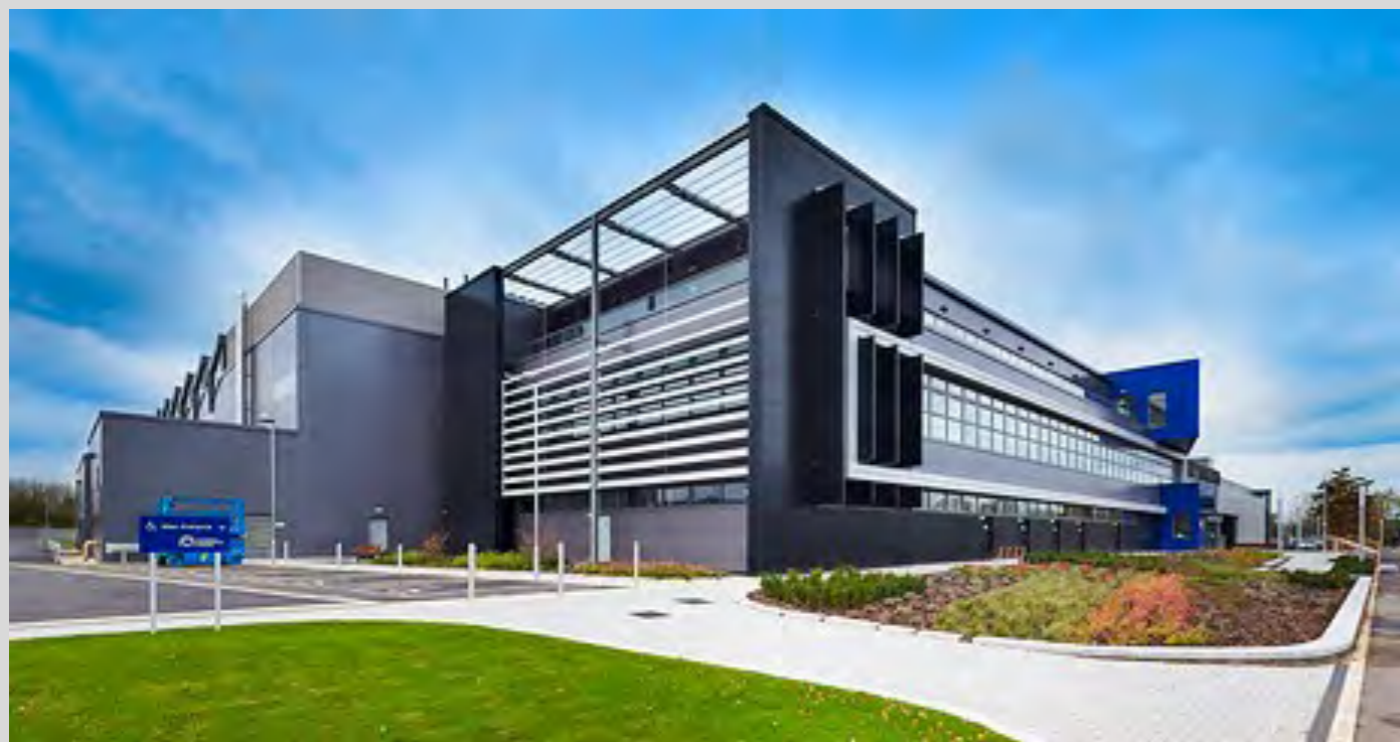
The National Composites Centre at the Bristol and Bath Science Park is a good example of a Research and Development complex with three storey 'active frontage' onto a spine street comprising ancillary offices and a legible entrance with a single storey 'supershed' concealed behind.
